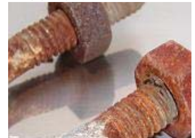
Rust and fixed bolts & nuts
