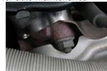
Rust and fixed bolts & nuts
