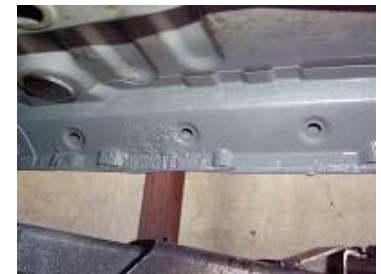
Anti-rust coating for welding
